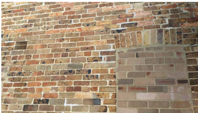
Figure 107: Brick infilled windows and different designs of metal ventilation grilles found on main facade facing Nimrod Street.
