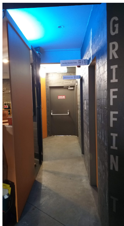
Figure 119: Corridor leading to amenities with door to rear lane at the end. Source: TZG Architects, 2022.
