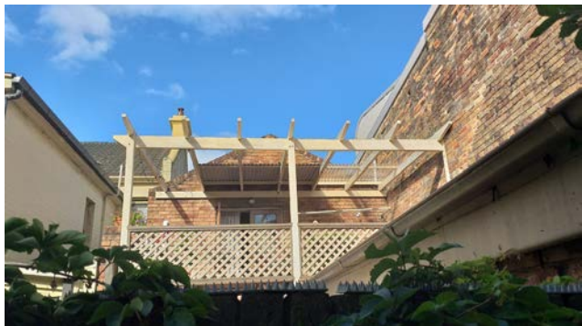
Figure 94: View of back of terrace house at 12 Nimrod Street from the rear lane. The external wall of the Griffin Theatre marks the perimeter of the property boundary.
