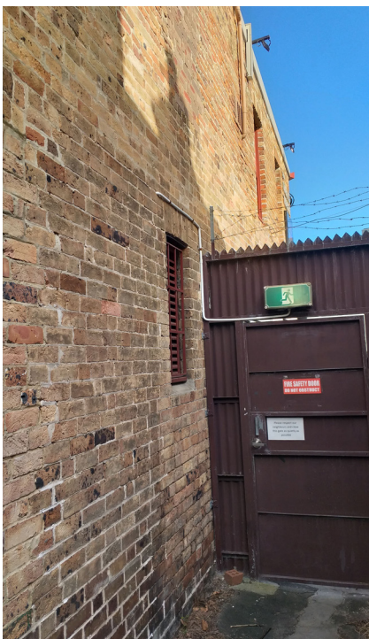
Figure 103: Evidence of repointing and brick repairs to facade of theatre in rear lane.
