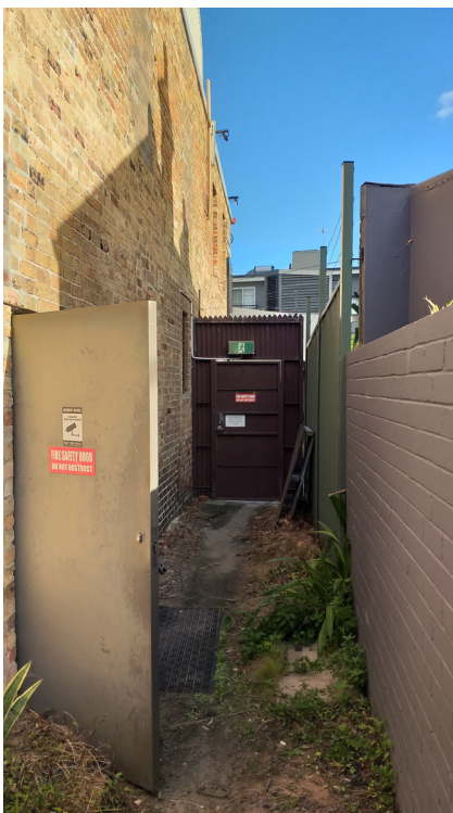
Figure 100: View of metal gate marking boundary to Nimrod Street. Internal access to rear lane is given at the end of corridor leading from main foyer (left).
