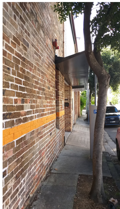
Figure 104: View along Nimrod Street of steel awning above the main entrance to the theatre.
