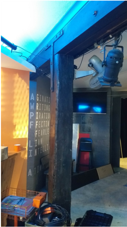
Figure 121: View of timber column and beam supporting the upper levels and separates the foyer and bar areas.
